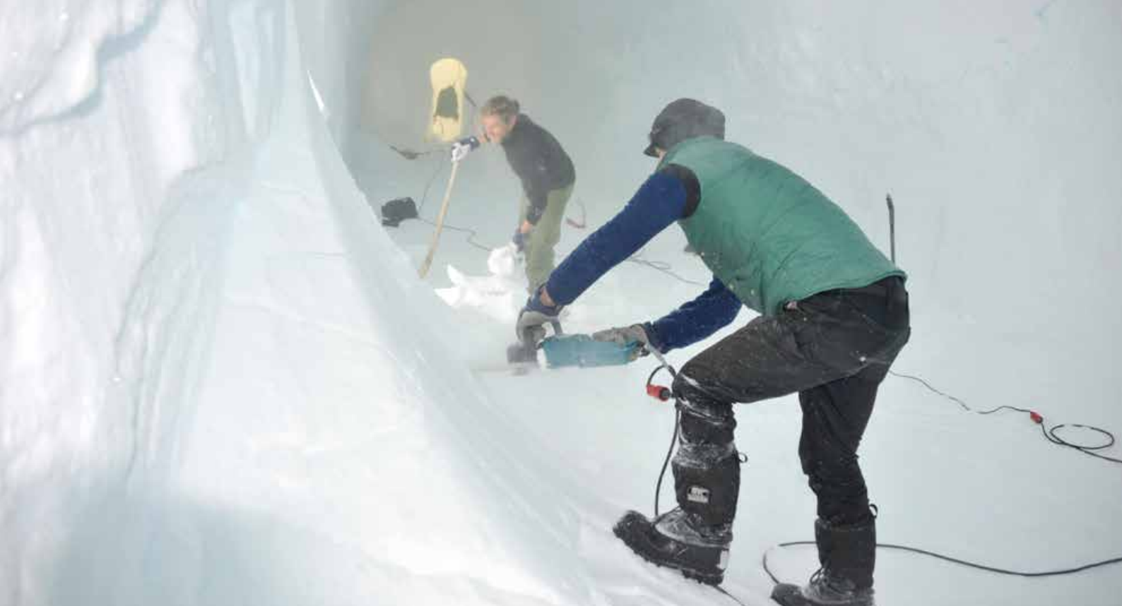
Equipped with a chainsaw and a shovel, the scientists are taking on the Greenland ice and building the EastGRIP tunnel system. Photo: Alfred Wegener Institute | Sepp Kipfstuhl
